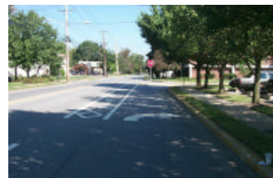
This intersection is properly striped, however many intersections do not meet national design standards
