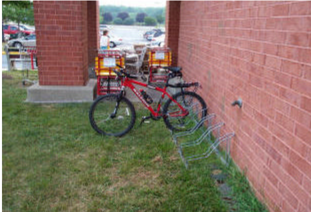
Acme Supermarket, Suburban Plaza. This is a good design, economical, and the lock can reach the frame, as seen in the picture right. As with any rack, it is imperative that the rider can lock the frame to the rack, as most bikes today come with quick release wheels/hubs.
