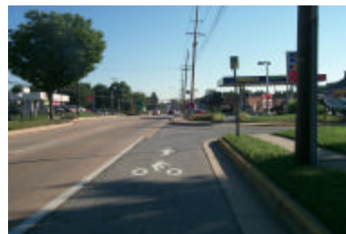
The bicycle lane on Elkton Road disappears in some locations
