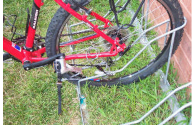
Note the lock around the portion of the frame just behind the pedal. Both a wheel and the frame can be easily locked with this design.
