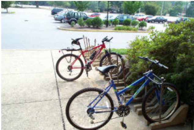
This is an older post design. Note the “trays” made of concrete, and the thinner posts.
