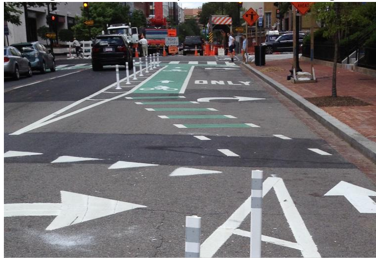
Photo 6: Green Paint across Mixing Zone on M Street NW in Washington DC
