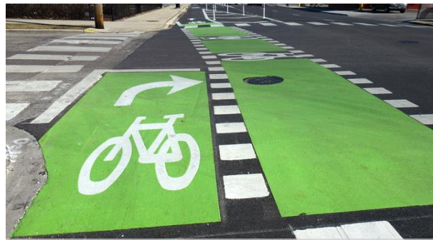
Photo 4: Two-Stage Turn Queue Box (Source: NACTO)
