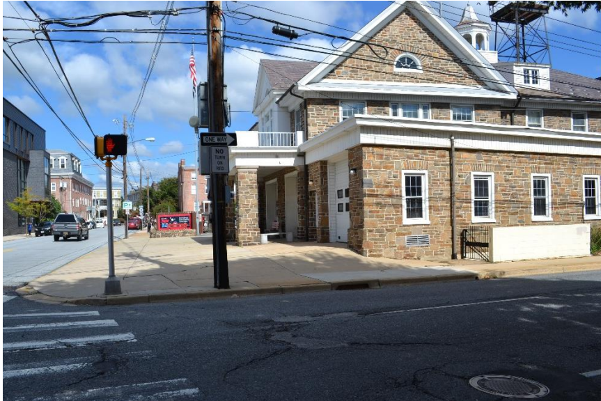
Photo 8: Aetna Fire Station
